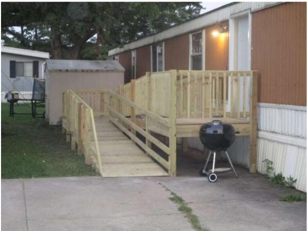
The second ramp was built in Normal, as well. This family had a very small ramp at their garage door but they were unable to use it.. too small and too steep. We were able to build a functional ramp with a proper slope so this family can get in and out of their home safely. Extra points and a thank you to Duane and Dennis!
